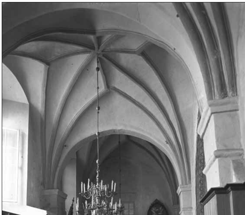
Fig. 8. Stellar vault at St Nicholas' Church in Pärnu. Photo by Armin Tuulse, 1943 (Art Historical Photograph Collection of the University of Tartu).
