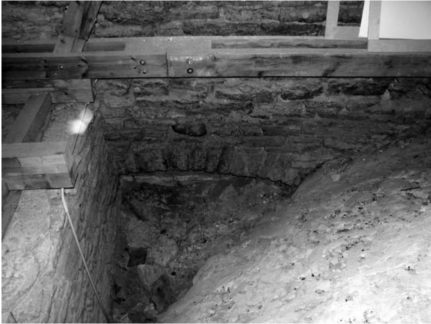
Fig. 7. Segment arch of the southern niche in the eastern wall of the nave seen above the chancel vault. Photo by Villu Kadakas.
