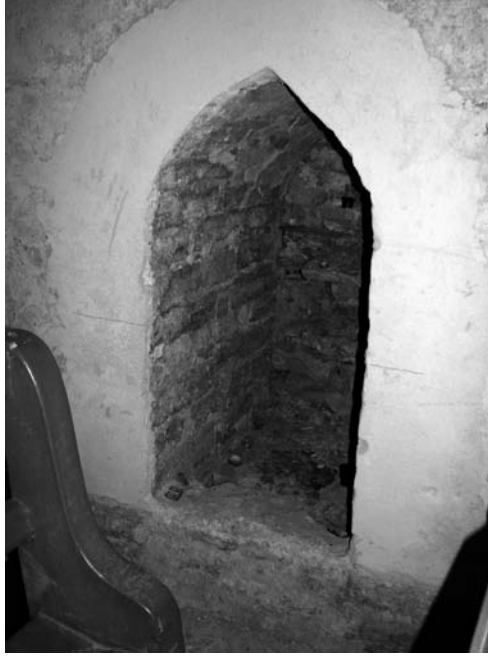
Fig. 6. Partly opened sacristy doorway. Photo by Villu Kadakas.
