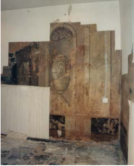
Fig. 5. Riga, 11 Kalku Street. Wall painting on plaster. Late 18th century. The painting was covered up before it was entirely uncovered. Photo by Juris Zviedrāns, archives of the Architectural Investigation Group Ltd.
