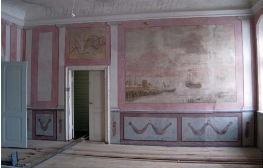
Fig. 3. Limbaži, 4 Burtņieku Street. Second floor colonnade painted on plaster, after conservation. The last quarter of the 18th century. Photo by Marina Mihailova, archives of the Architectural Investigation Group Ltd.
