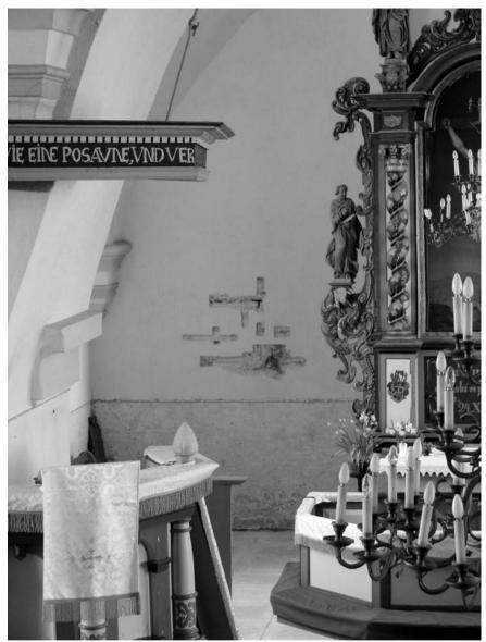
Fig. 4. Discovering the aumbry niche in the eastern wall of the chancel - plaster partly removed from the masonry (in the middle of the photo). Photo by Villu Kadakas.
