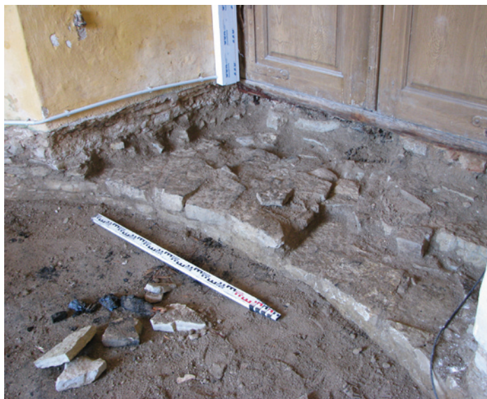
Fig. 6. Round foundation of Paide church tower.
