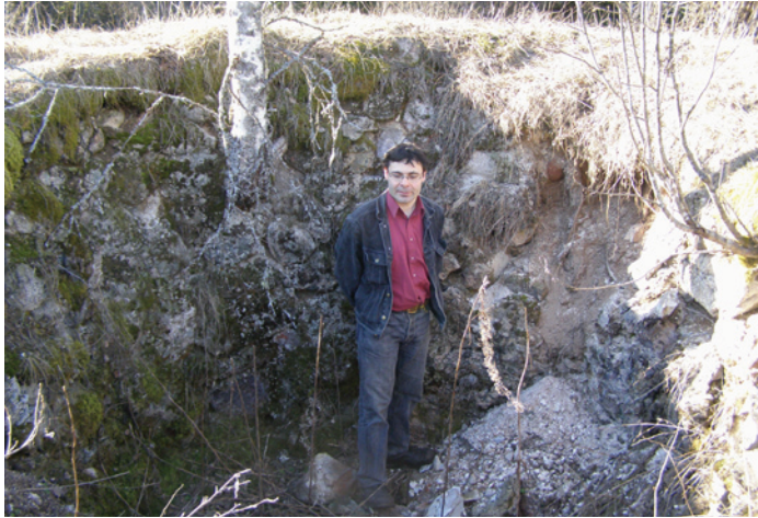
Fig. 5. Stone inner lining of a limekiln in Jõune village prev. Tolli farmstead.
