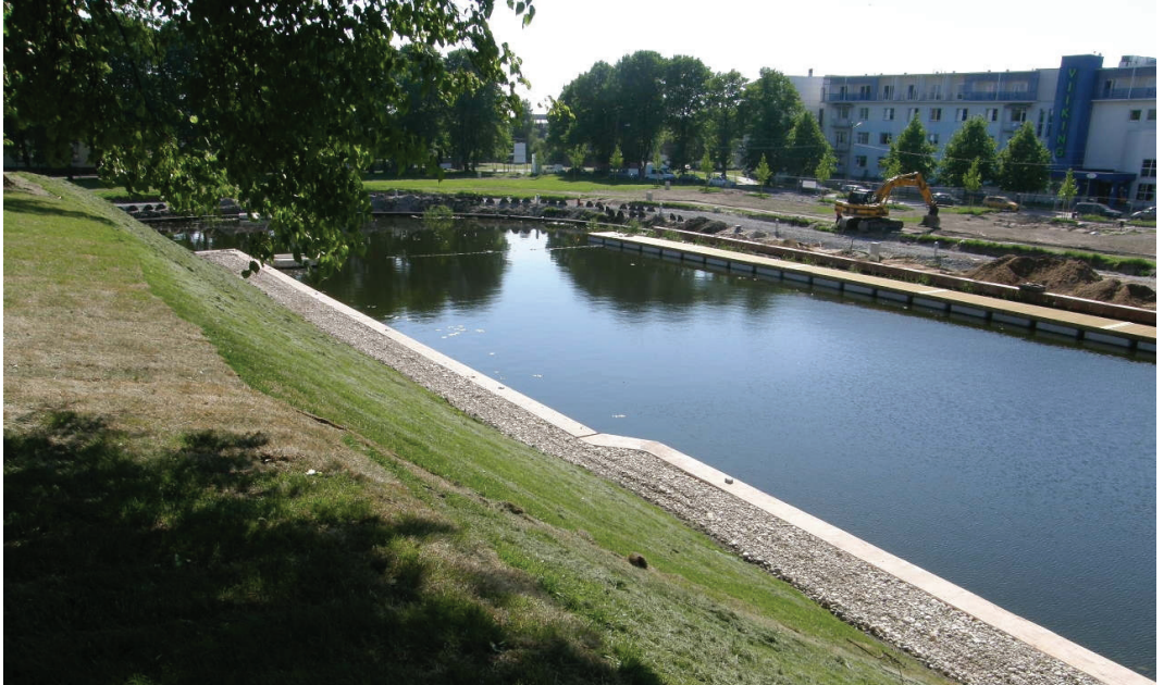
Fig. 3. New construction at the waterline shifted away from the wooden constructions by the western side of the bastion Luna.
