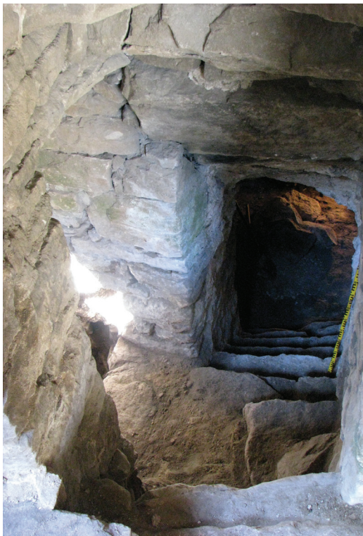
Fig. 8. The reopened stairway from the cellars of the gate tower to the western courtyard.
