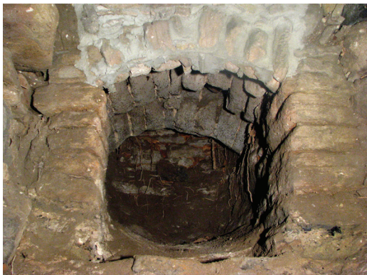
Fig. 9. Hypocaust oven between the two westernmost cellar rooms of the gate tower.
