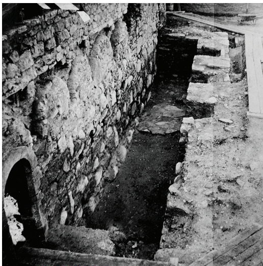
Fig. 5. Area of the western cloister excavated in 1961: to the left the eastern wall of the western range with restored niches for cloister vaults, to the right remains of the eastern wall of an older building, on top of which a wall or pillars of the later cloister were set.
