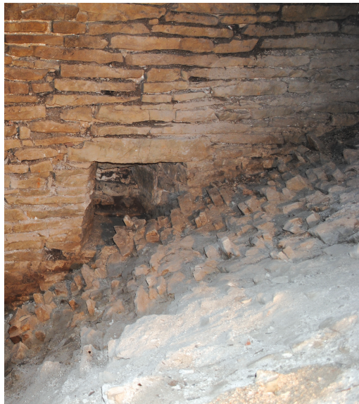
Fig. 2. One of the windows that had been partly walled in with the construction of the arches, found in the eastern wall of the church.
