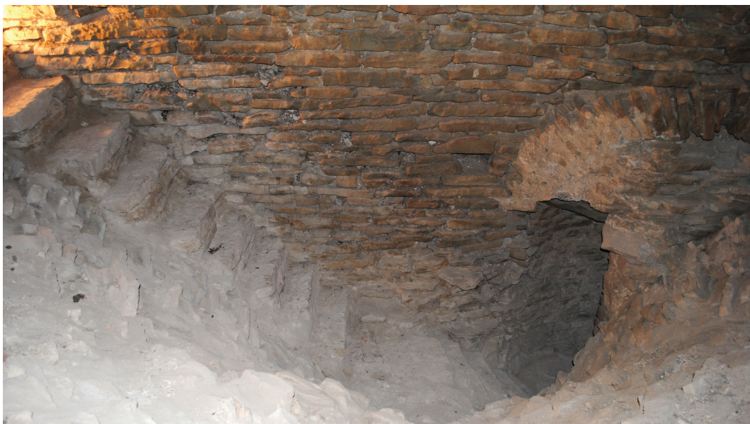
Fig. 3. The excavated passageway and stairs leading on top of the arches in the northern wall of the church.
