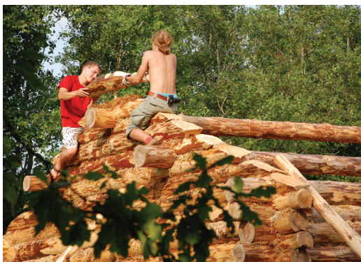
Fig. 7. Assembling the support construction of the roof.
