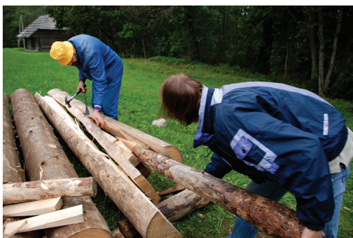
Fig. 4. Making wedge-split boards.
