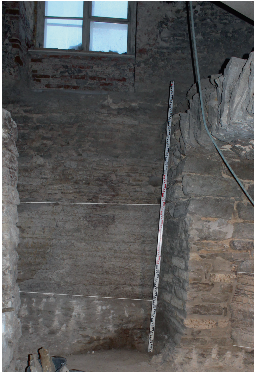
Fig. 6. View towards the edge of the plateau. The edge of the quarry forms a natural ‘wall’ with weathered edges. During building works, 60 cm of limestone was removed from the old quarry floor.
