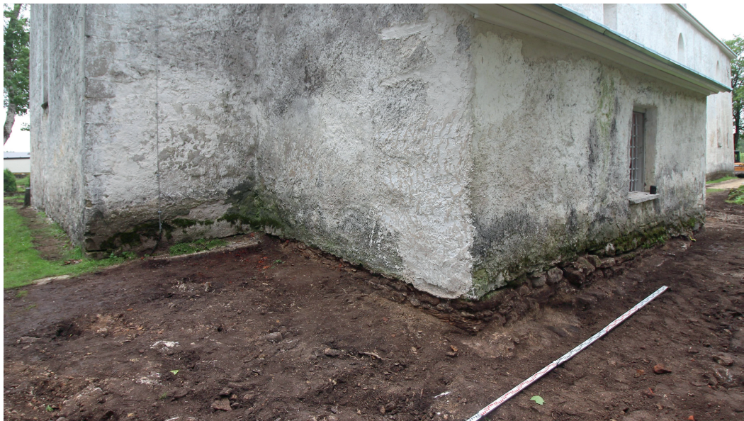
Fig. 7. A protruding edge of foundation on the northern side of the sacristy of the Järva-Jaani church.
