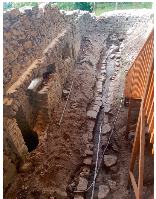
Fig. 6. Sewage and rainwater conduit in the Padise Monastery.
