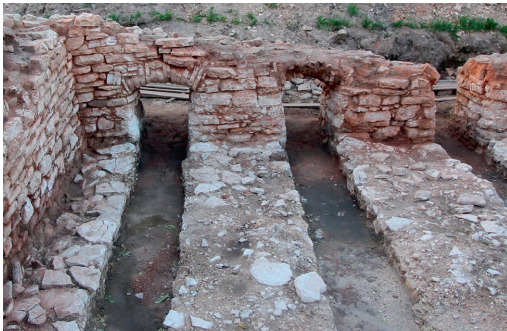
Fig. 9. Inner view of the façade of the lime kiln with arched entrances.
