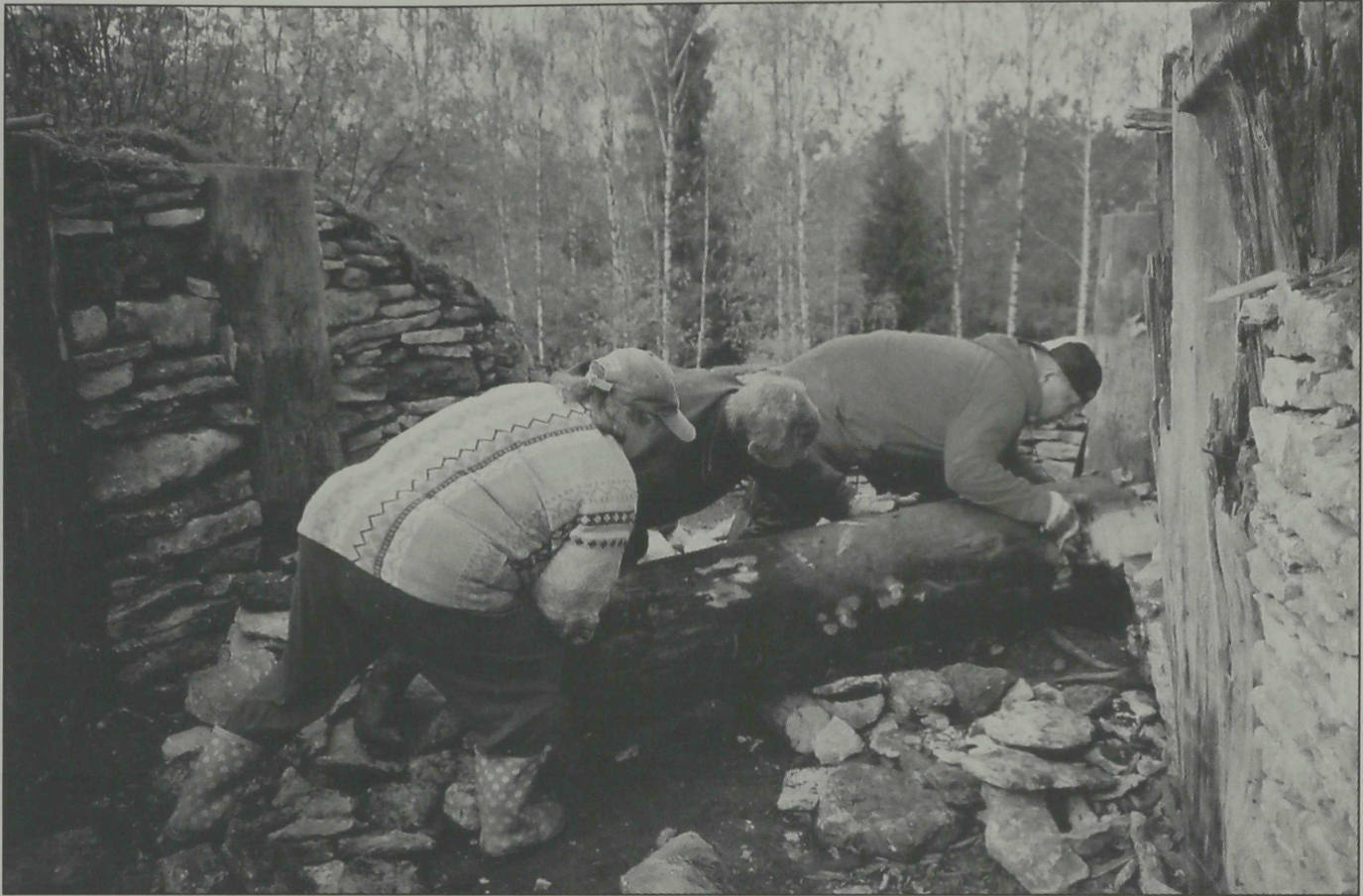
Fig. 6. Placing a new post into the post-hole. View from East. Jn 6. Uue posti asetamine postiauku. Vaade idast.
