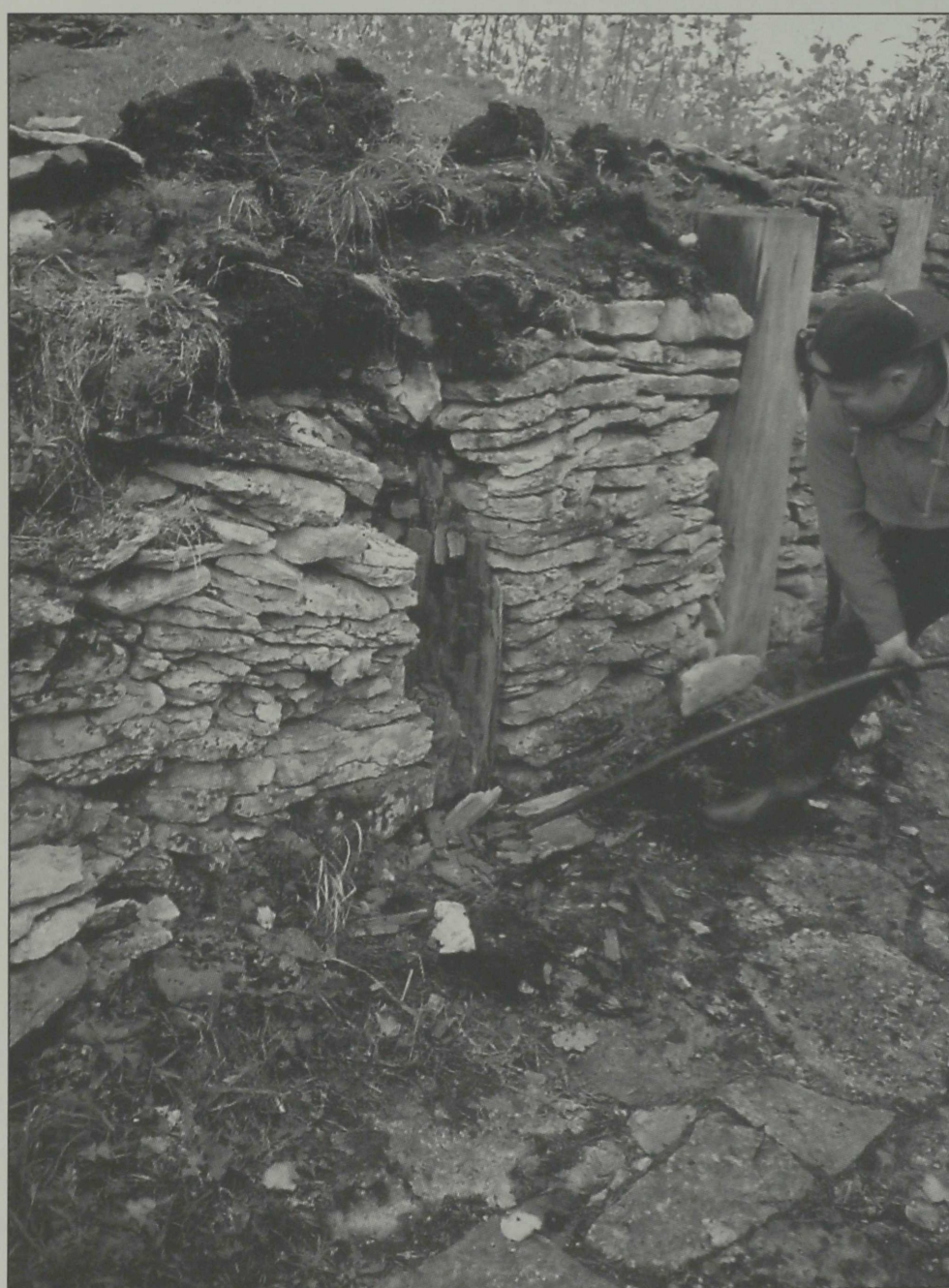
Fig.5. The removal of the first decayed post in 2006. Jn 5. Esimese kõduposti eemaldamine 2006. a.
