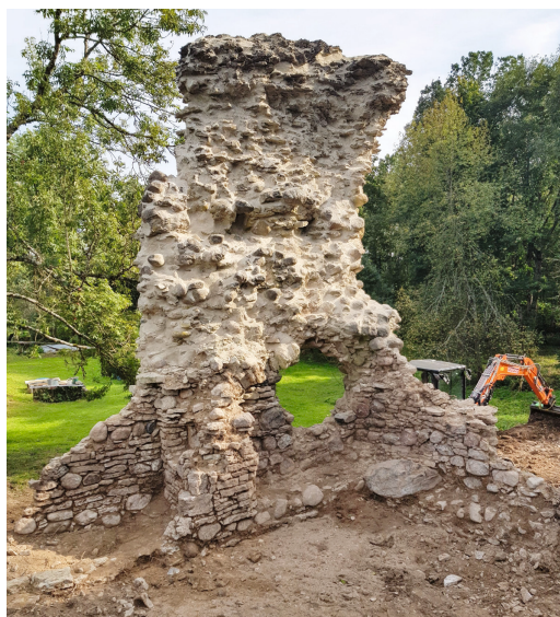
Fig. 7. Ruins of the medieval manor house of Angerja, south-eastern corner after excavation. Remains of a portal and stairs to the basement (left) and a wall niche with a segment arch (right).
