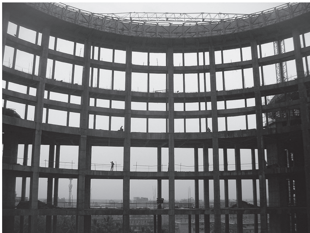
Photo 1. Temple of the Vedic Planetarium under construction. Photo by Marje Ermel.
