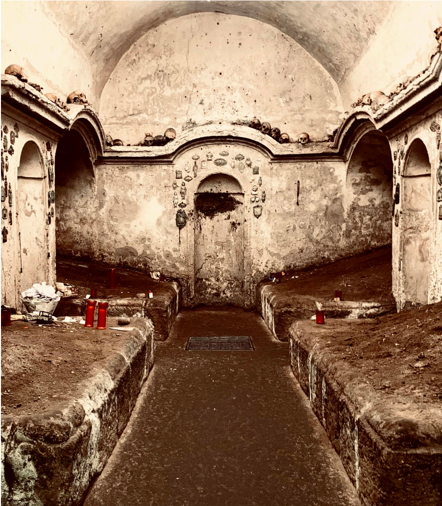
Figure 1. Typical structural organization of a terrasanta : a vaulted room with four “giardinetti”, a central corridor and niches; above the latter a ledge for the laying of the skulls runs along the walls; in the middle of the corridor one can see the grate that gives access to the ossuary below. (Church of Santa Luciella, Naples)
