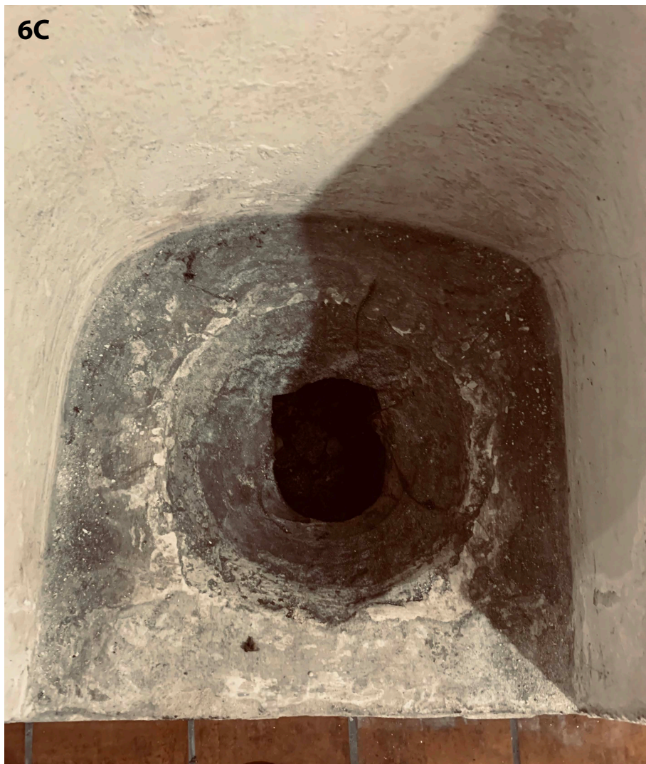
Figures 6. A row of sitting scolatoi within niches along the hypogeum wall (A, B) equipped with a seat with a hole in the centre (C). Between a niche and another, there are metal attachments (B, arrows) for an object (probably a rod or a rope) that was supposed to prevent the corpses from falling forward. Evident signs of recent restoration interventions are detectable in this room. In particular, the drainage system used for the outflow of cadaveric liquids is no longer detectable. (Church of San Severo al Pendino, Naples)
