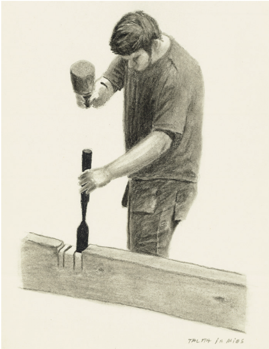
Figure 1. A carpenter is using a slick to finish a notch cut with a chainsaw. The slick has a strong wooden handle and can also be used to pull and break things to some extent. The man is standing in a well-balanced position, his legs slightly apart, left foot a little forward. The bottom of the notch is located rather low, but the slick is long so that the end of the slick handle is at a height where the man does not have to lift his arm higher than his shoulder when he hits the slick with the club. The club hits the head of the slick at elbow height. The height of the log is also suitable for cutting out the lateral groove, but too low for smoothing the bottom of the notch with the slick. The man probably gets down on his knees to 'adjust the height' so he can work on the bottom of the notch.
