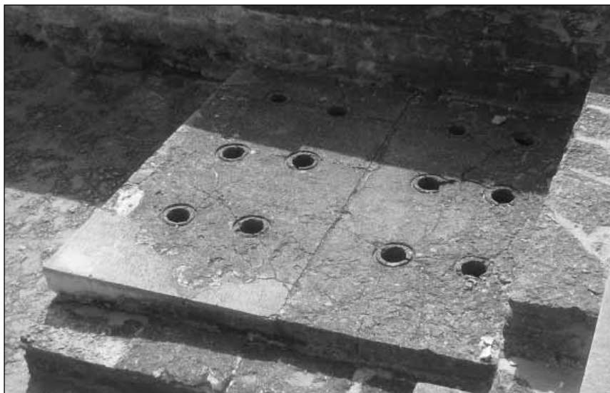
Fig. 8. Hot plate of a heat storage hypocaust in the Pirita Convent of the Brigittines. Photo by Andres Tvauri.
