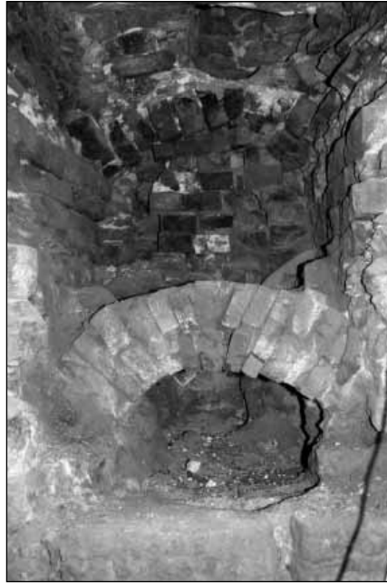
Fig. 5. Heat storage hypocaust found in a room under the dörnse in Tallinn Pikk Street 34 in early spring 2009. Photo by Andres Tvauri.
