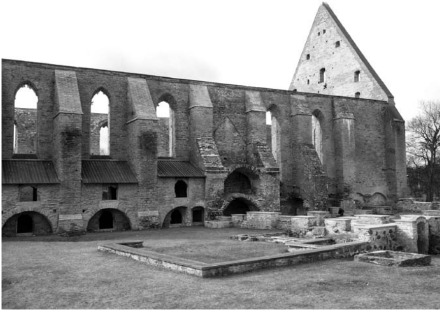
Fig. 20. Excavated and conserved foundations of the abbess's residence. Photo by Heidi Tooming.
