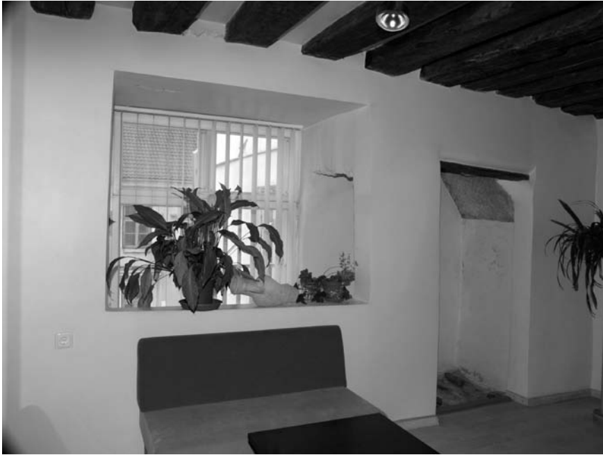
Fig. 18. Niche in the northern wall, later turned into a window. Photo by Heidi Tooming.
