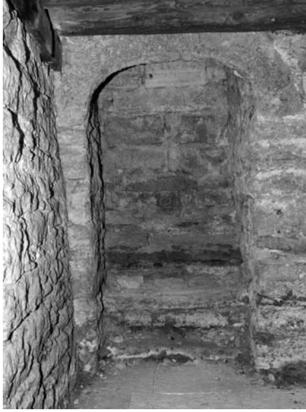
Fig. 4. Old, walled-up basement staircase. Photo by Heidi Tooming.
