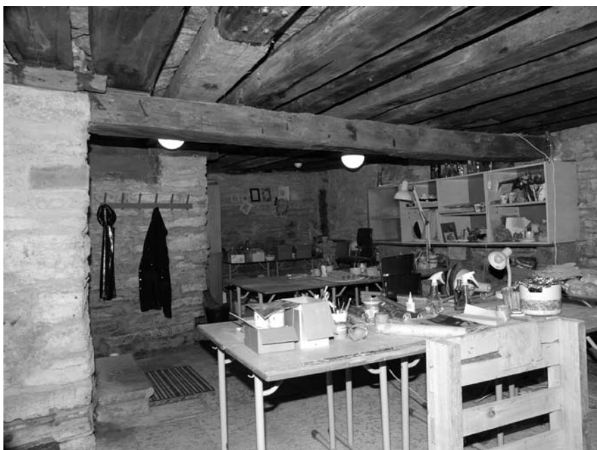
Fig. 12. Ceiling beams in the southern basement. Photo by Heidi Tooming.
