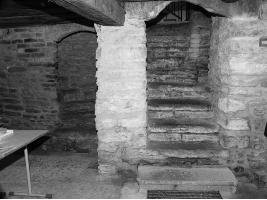
Fig. 7. Stairways in the northern wall of the southern basement. Photo by Heidi Tooming.
