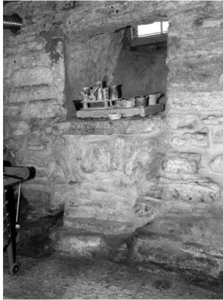
Fig. 10. Inlet of the water channel and a window in the western wall. Photo by Heidi Tooming.
