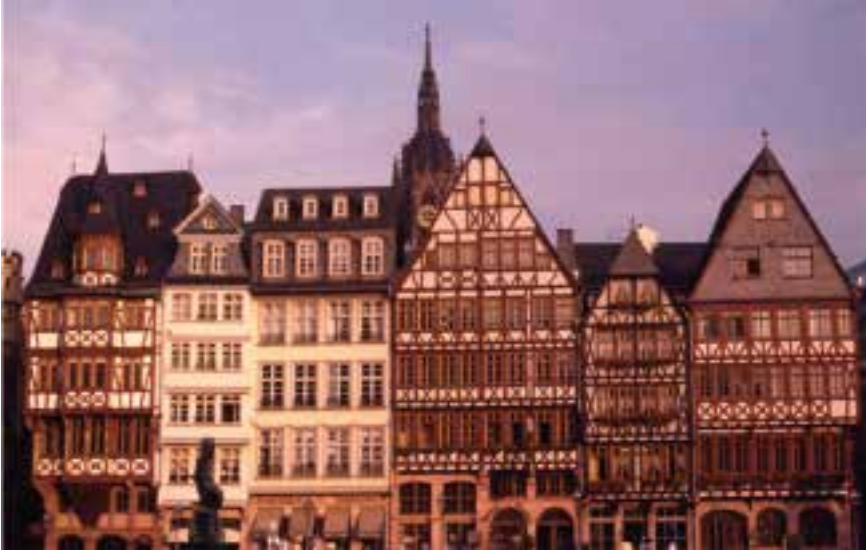
Fig. 11. Frankfurt – Römerberg, reconstructed medieval buildings after bombings of the Second World War (photo Kaisa Broner-Bauer)
